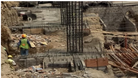
Gambar 3. Pile Cap As 4B
