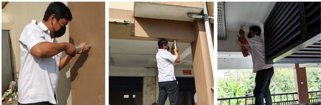
Figure 8. Hammer Test Tests on Columns, Beams and Plates of Rusunawa Building
