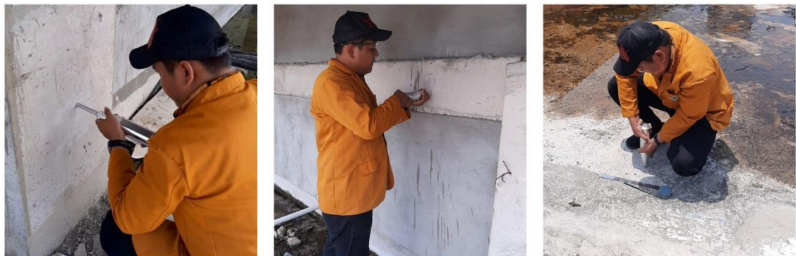
Figure 4. Hammer Test Tests on Columns, Beams and Plates Meeting Building
